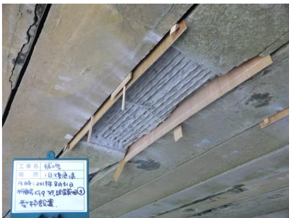
[写-6-9 型枠設置状況]
